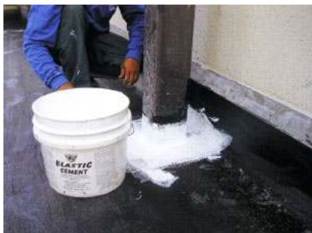
Application of Membrane
