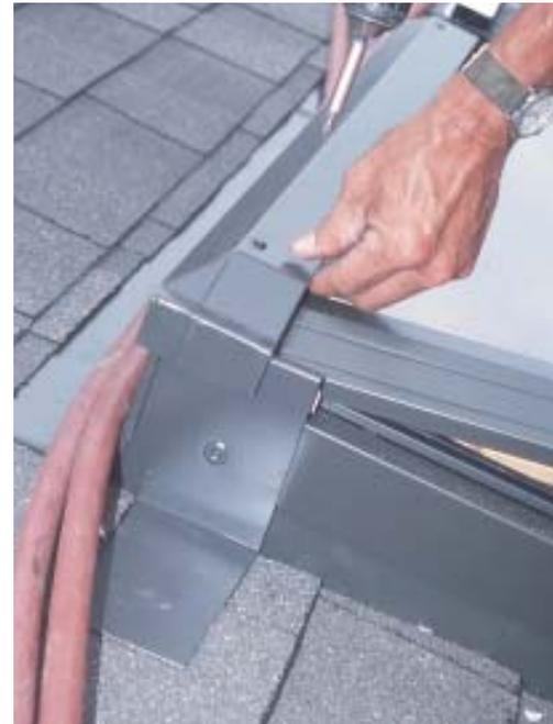
**Figure 10.** Reinstalling the skylight's cladding completes the process. The bottom goes on first (top left). Slots in the bottom receive the side pieces (top right). Plastic inserts in the sides receive the screws inserted through the head flashing (above left). Finally, the top cladding piece is slipped over the head flashing and secured with two screws (above right).
