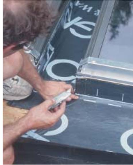
**Figure 6.** The top piece of membrane laps over the sides (left), and a slit cut outward forms a flap that folds around the corner (right). The membrane's leading edge is adhered to the roof deck under the felt.
