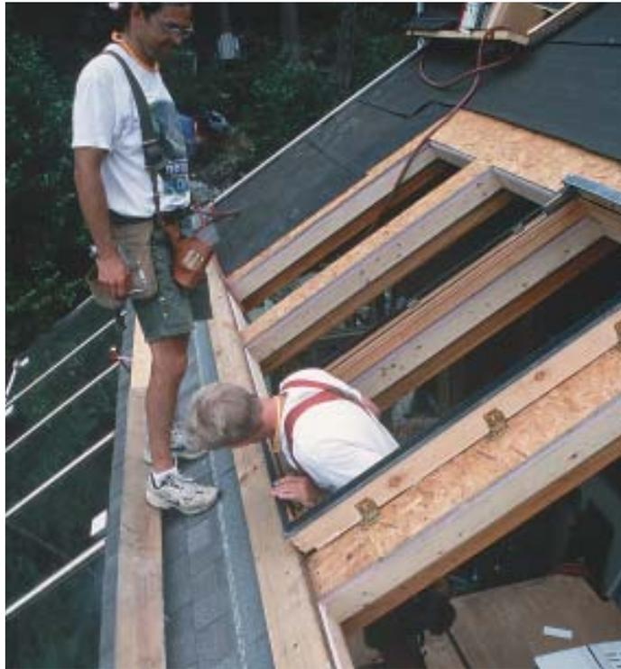
**Figure 3.** Tacking a 2x4 cleat to the sheathing keeps units in a straight line and prevents them from sliding off the roof. Once the units are secured, the cleat will be removed so shingling can continue.
