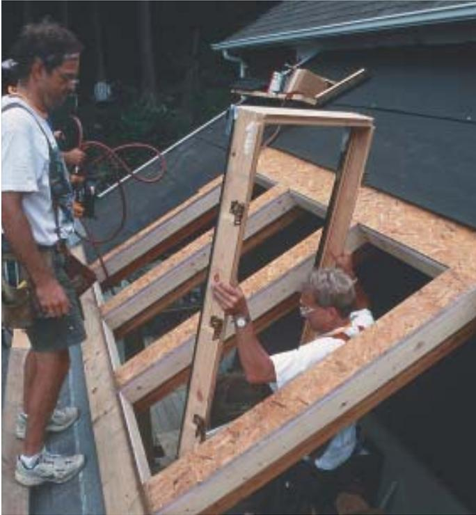
**Figure 1.** Removing the sash makes handling safer and easier. Narrow strips of ceiling between skylights make layout mistakes really obvious, so special attention is given to accurate spacing during framing.
