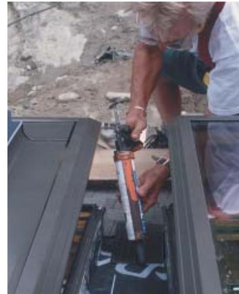
**Figure 7.** When the shingling reaches the skylight, the sill flashing is slid up from the bottom and fastened at the top corner with the manufacturer's special nails (left). The first piece of step flashing overlaps the sill flashing  $3\frac{1}{2}$  inches. Where adjacent sill flashings overlap, urethane sealant provides extra insurance against leaks (right).
