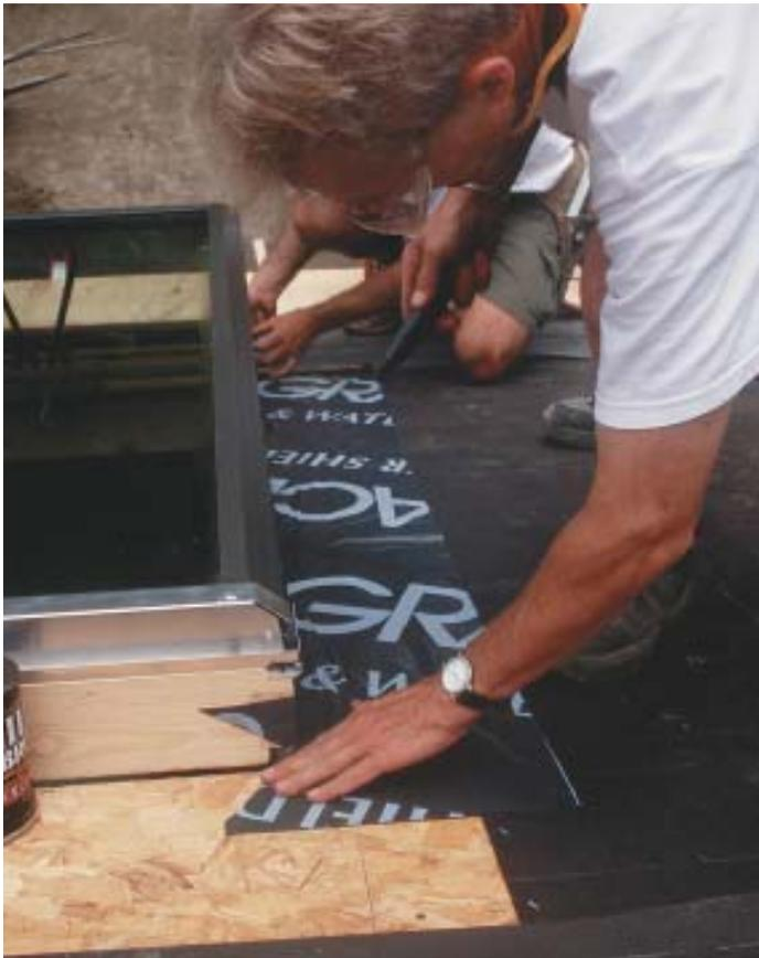
**Figure 5.** To reduce the chance of leaks, the author uses a single piece of membrane in the space between skylights. Folding the membrane in half helps to keep it from sticking to itself (top left). Aligning the membrane's edge on the first unit and smoothing toward the roof deck and back up the second unit minimizes wrinkles (top right). Cutting the corner allows the vertical leg to wrap around the top corner (above).
