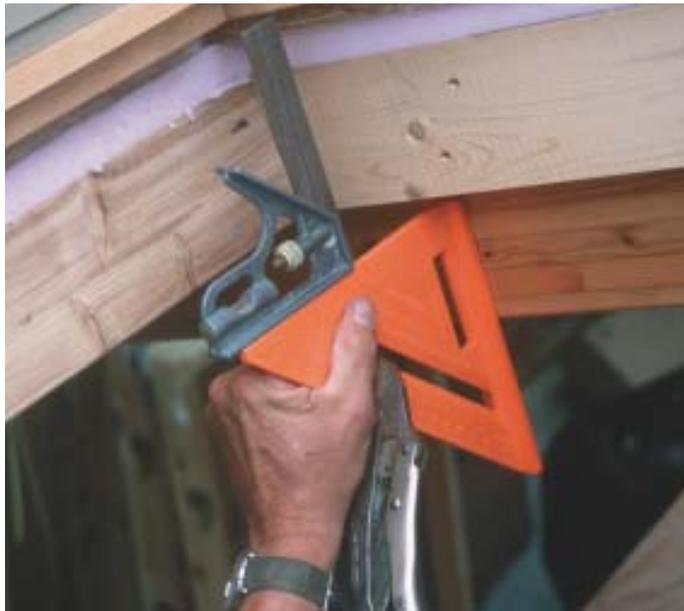
**Figure 2.** An improvised tool helps center the unit in the opening. The speed square rides along the rafter, and the combination square indicates the space between the unit and the rough opening. Note the layer of polystyrene insulation installed beneath the roof sheathing.
