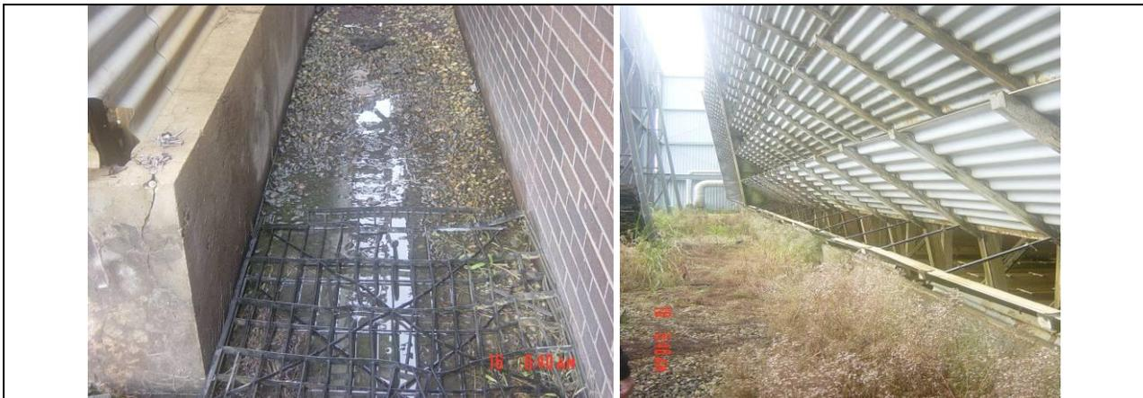
The pictures show the accumulation of water from a leaky basin.
