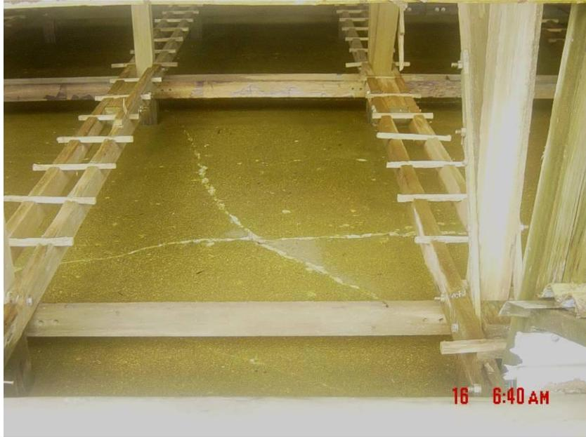
An illustration of deterioration and discoloration due to long term exposure to dilute sulfuric acid in the water treatment system.
