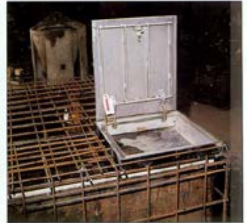
Frame depth designed to match slab thickness
