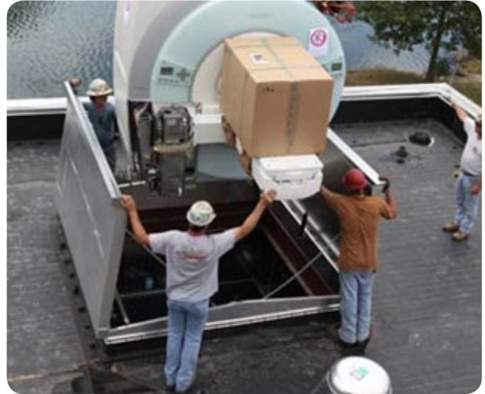
Equipment Installation Application
