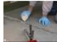
5. Soak sand with Slabweld until saturated leaving a slight hump.
