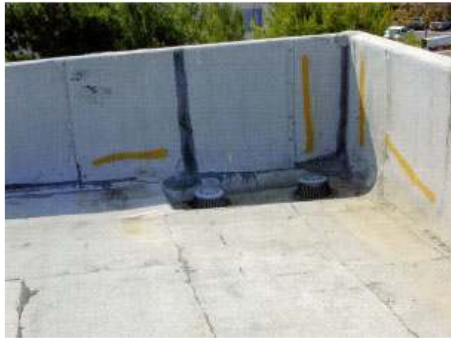
Reflective Surface Coating is Applied
