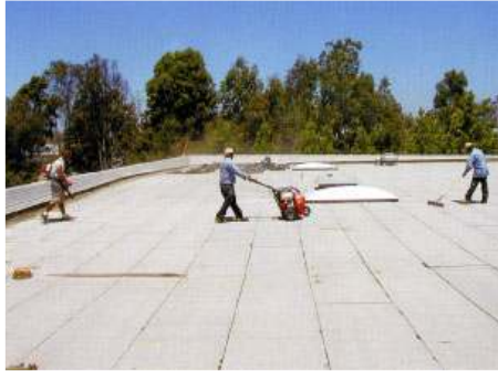
Clean & Prep existing roof
