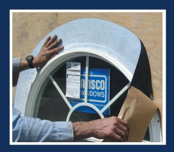
Protecto Flex® is a 90-mil thick peel and stick flashing tape. The flexible cross-laminated top surface will expand and conform to irregular or curved surfaces while the aggressive adhesive forms a permanent bond between the window fin and the building substrate. Protecto Flex gives you a total air and water seal without having to cut and patch in the membrane to conform to irregular or curved window and door openings.
