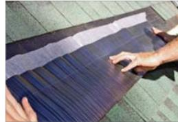
middle through the end cap. Roll out vent and pull tight; nail at 10 feet and again at the end of the roll.
