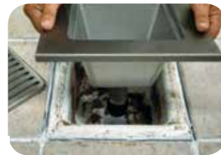
Insert stainless steel liner
