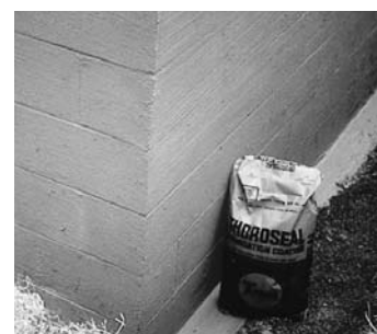
Sealed and waterproofed.
