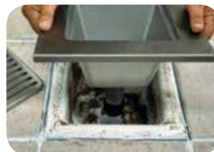
Insert stainless steel liner
