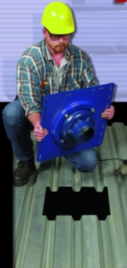
Preassemble Drain Body To Deck Plate
